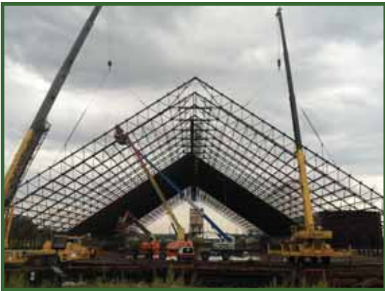
Brother Weldon Messerlie operates a 75 ton Grove and Brother Tyler Hickson operates a 35 ton Grove while taking down a grain storage building for Klinger in Sioux City
